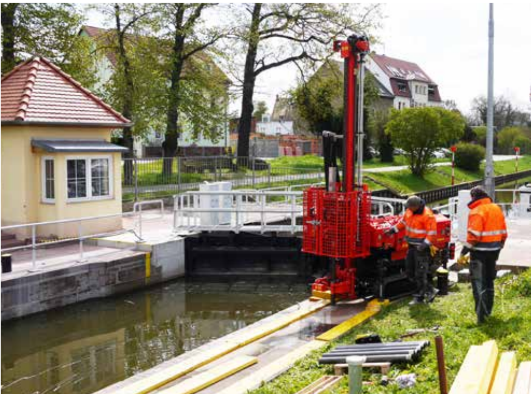
Core drilling at a canal sluice
