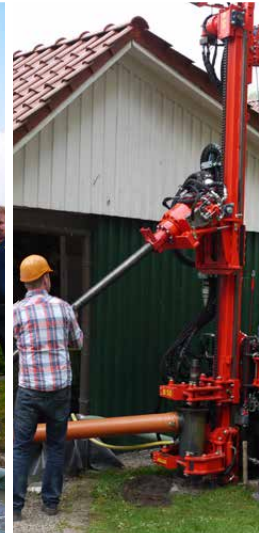
Rod replacement during flush drilling procedure
