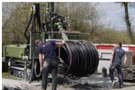
Installation of a geothermal probe
