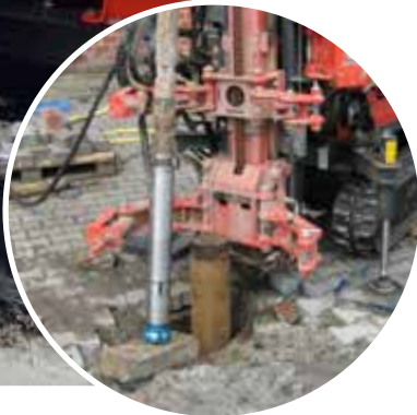
3" down-the-hole-hammer with drill crown
