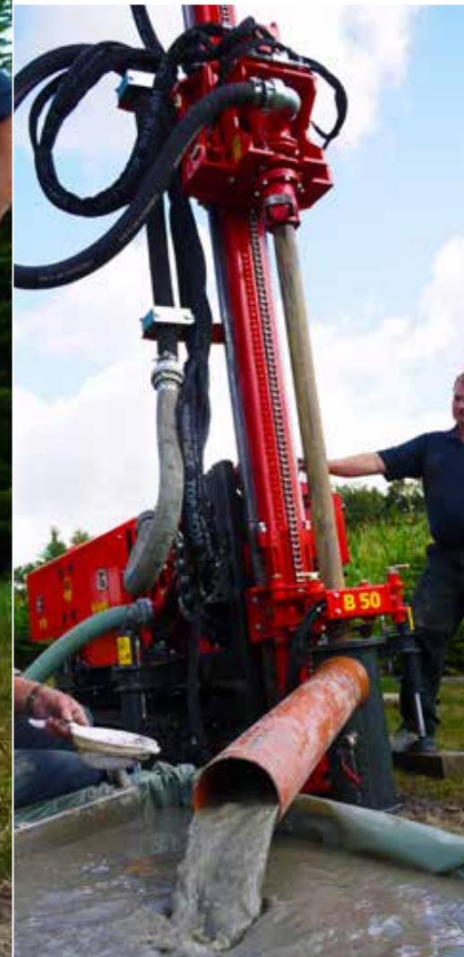
Sampling of material from the flush drilling water
