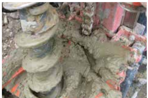
Drilling debris removed by the auger
