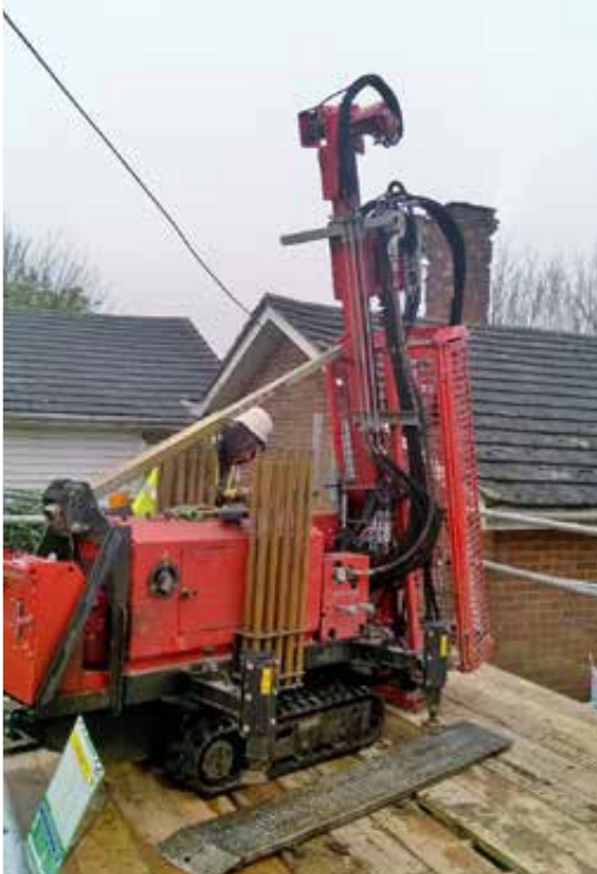
Probing to locate cavities.
