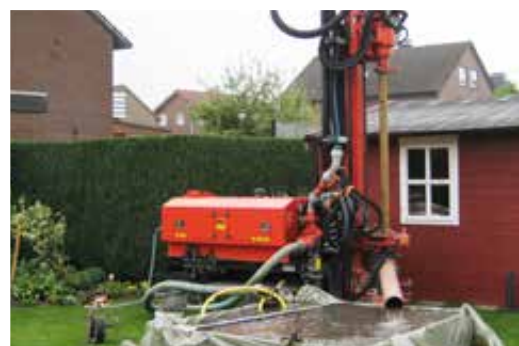
Well drilling in a fully landscaped garden
