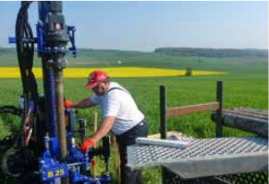
B 25 drill rig in use pulling cores
