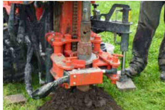
Hollow stem auger guided by the lifting clamp
