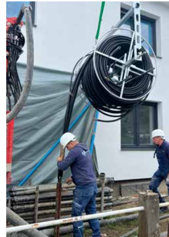
Reel enables safe and efficient insertion of the probe into the borehole
