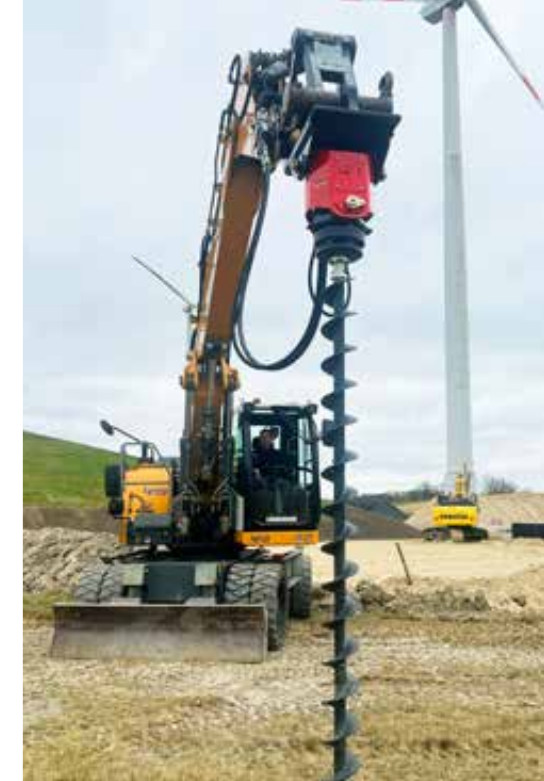
The EHD drive in use with a continuous flight auger for unexploded ordnance (UXO) detection
