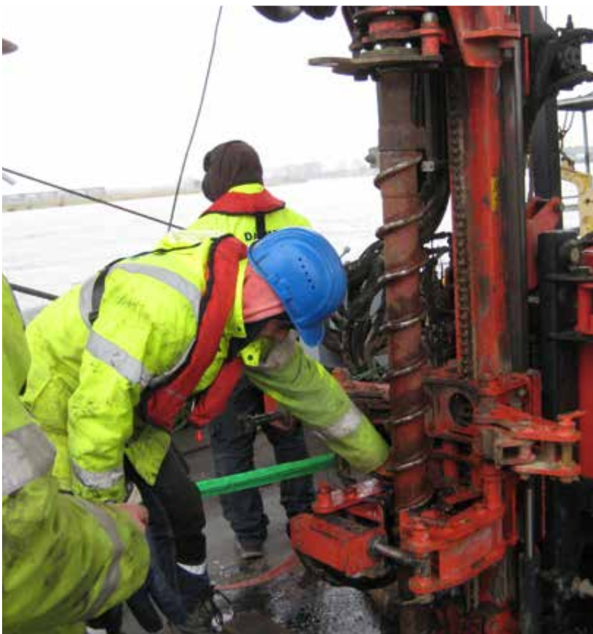
Probing using the hollow stem auger on a pontoon on the River Rhine
