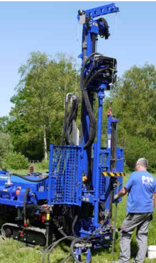
Dynamic probing with the ADLER-drill rig B 50
