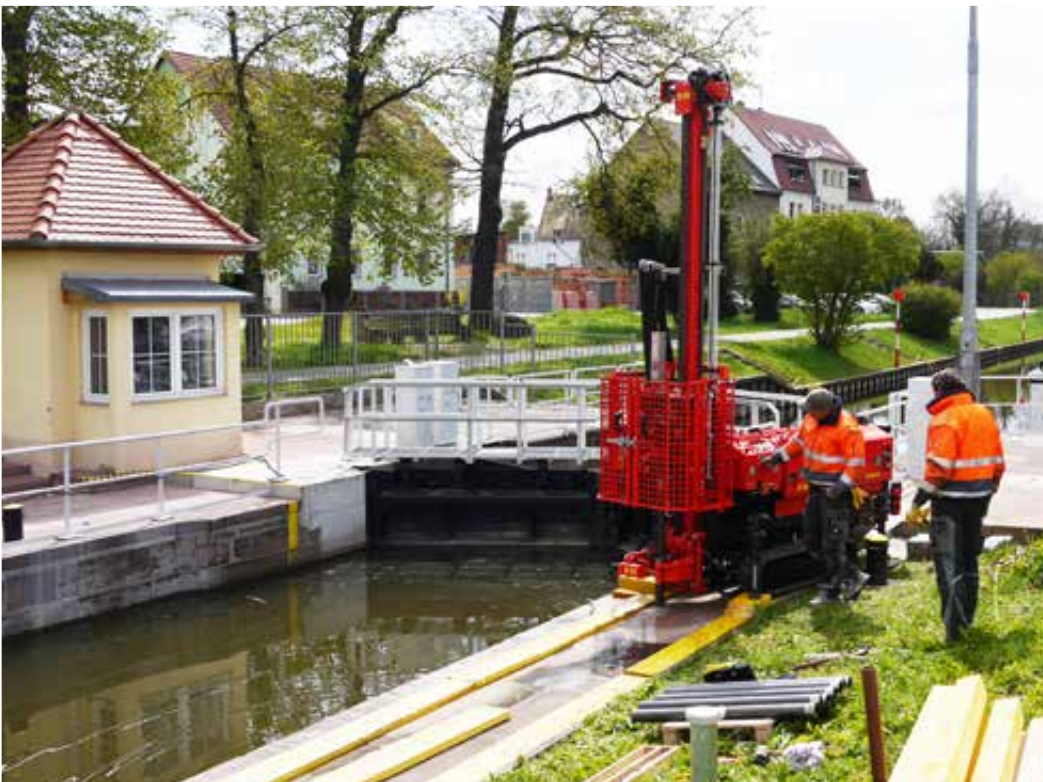
Core drilling at a canal sluice
