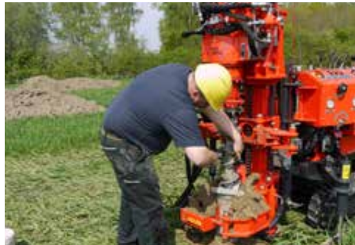
Dry drilling with external support casing
