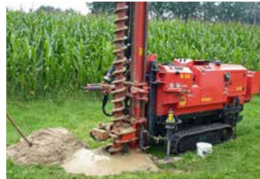
Working with the hollow stem auger
